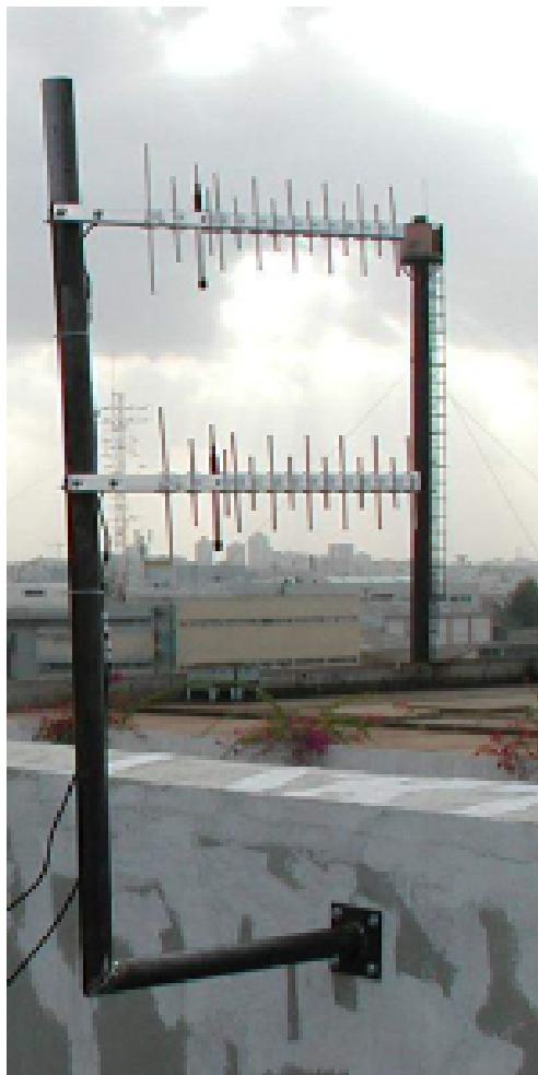
Figure: Example of Correct Installation of Directional Antennas
